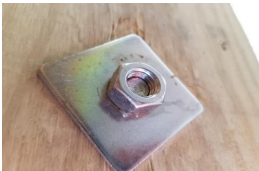
Bolt only just on thread of nut!
